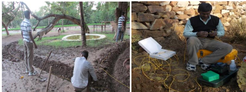
Fiber Optic Sensor Cable Deployment at Chhatbir Zoo & Panna
